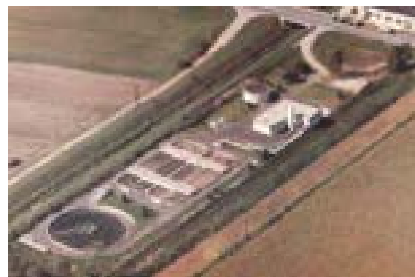
WTP & Other Corrosive Conditions
